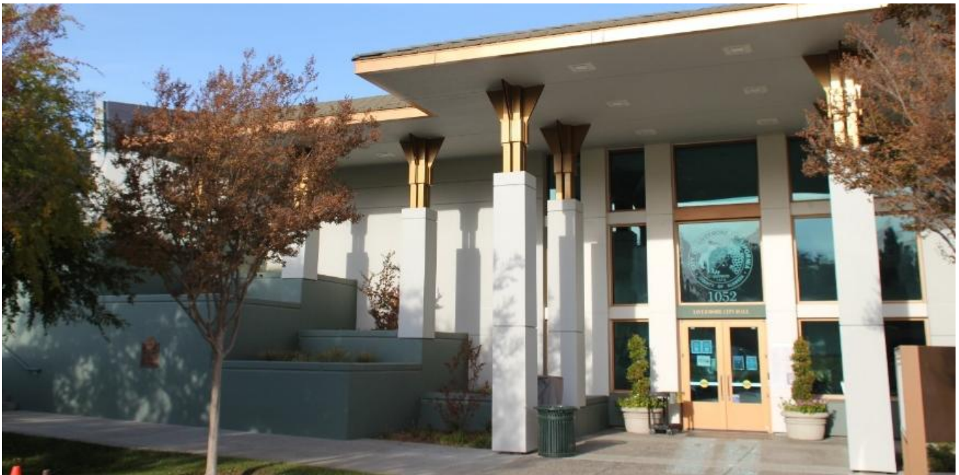
The City of Livermore plans for infrastructure upgrades and improvements using clear schedules, cost estimates, and allocating funding in the City's financial plan.
